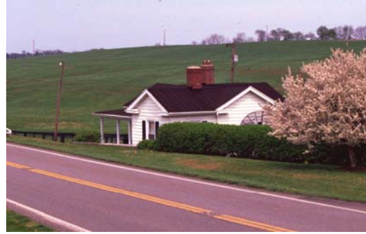
Figure 12. Toll house of Paris-Winchester turnpike, 2 miles from Concord Church (photo 1999).
