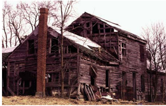
Figure 10. “Building out” as the family expanded: Jeremiah Duncan homestead, central two-storey log pen with log wing on right (c. 1790) expanded with frame ell on left, all covered with sawn siding from Brutus’ mill (c. 1840).
